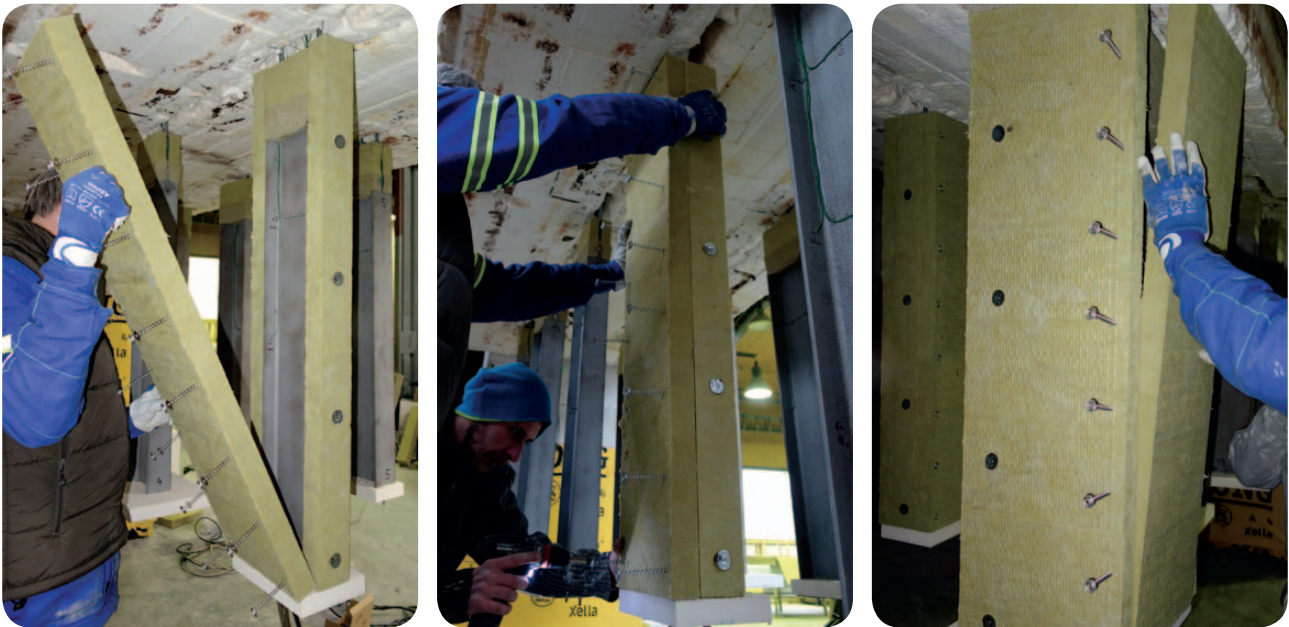
Fig. 6 Both methods can be also combined – important is to keep the distances (between pins 300 mm and between Fire Screws 150 mm)
