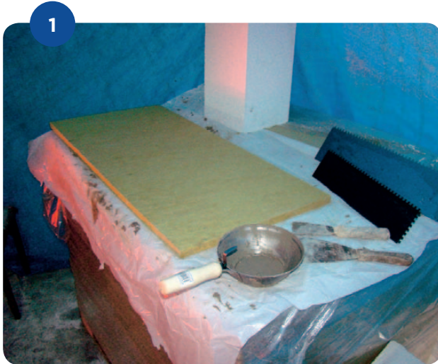
Inspect the slab and the tools used
