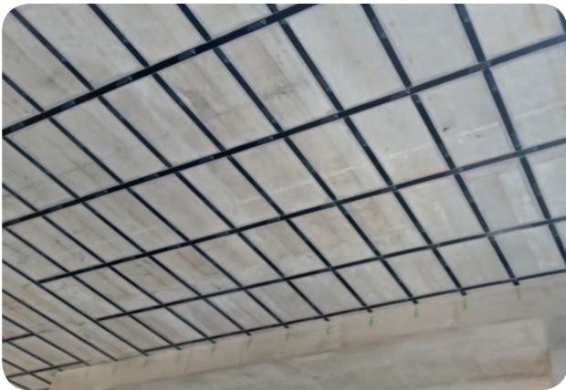
Fig. 17 Carbon fiber reinforced lamellas before fire protection
