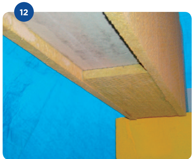
The flange is glued in the end
