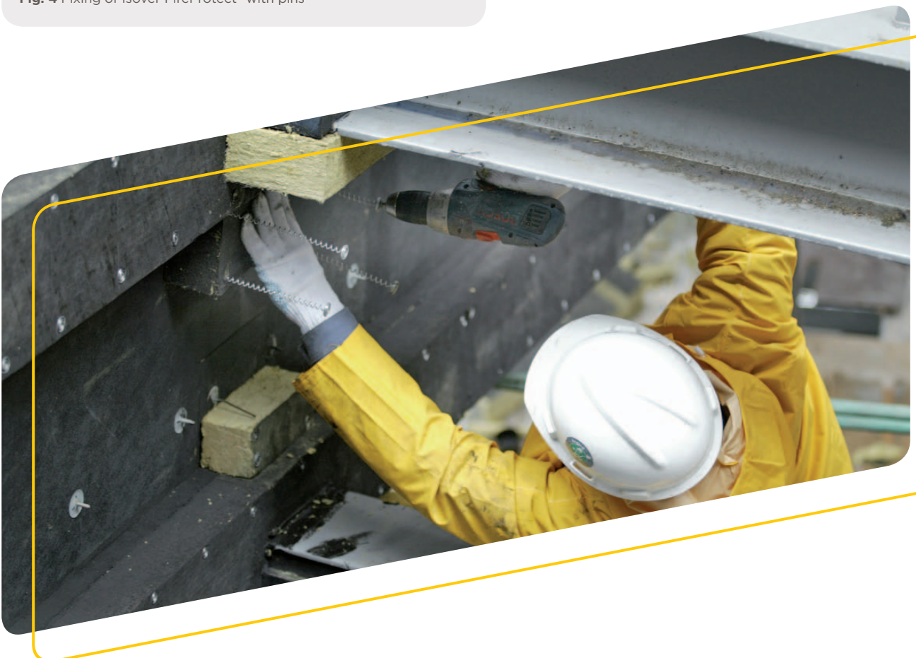
Fig. 4 Fixing of Isover FireProtect® with pins
