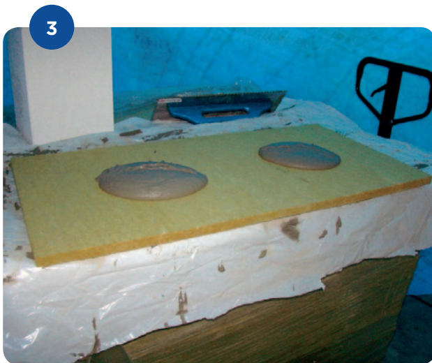
Apply an adequate amount of the adhesive on the slab
